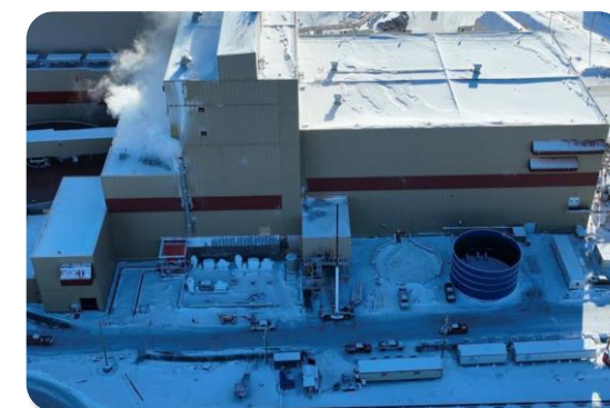
Structural work - North
