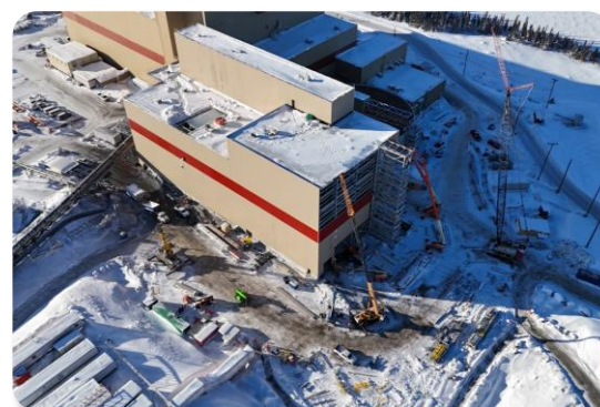
Structural work - South
