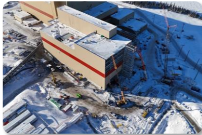
Structural work - South
