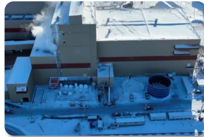
Structural work - North
