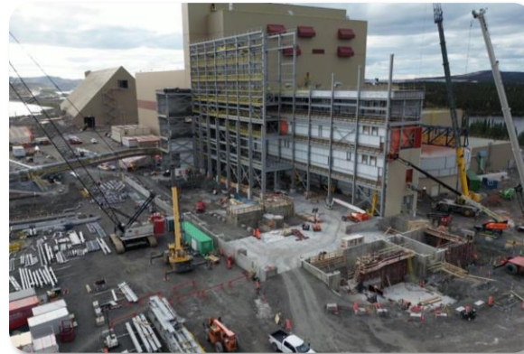
Structural work - South
