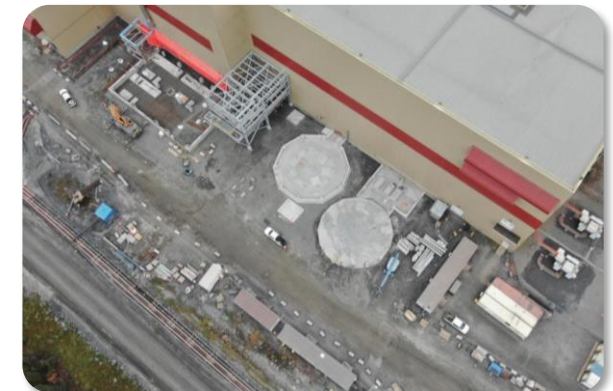
Foundation work - North
