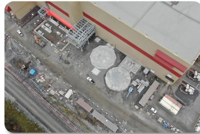
Foundation work - North
