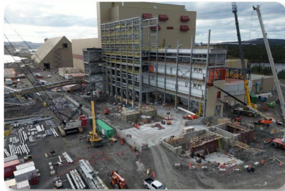
Structural work - South
